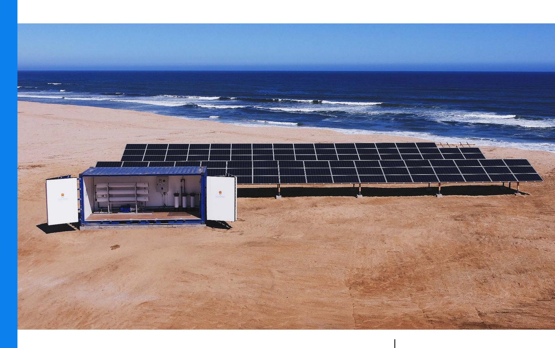
CASE NAMIBIA: THE SOLAR-RO SYSTEM UP-AND-RUNNING AT THE NAMIBIA UNIVERSITY CAMPUS, PRODUCING CLEAN WATER FROM THE ATLANTIC OCEAN., POWERED BY SOLAR.
